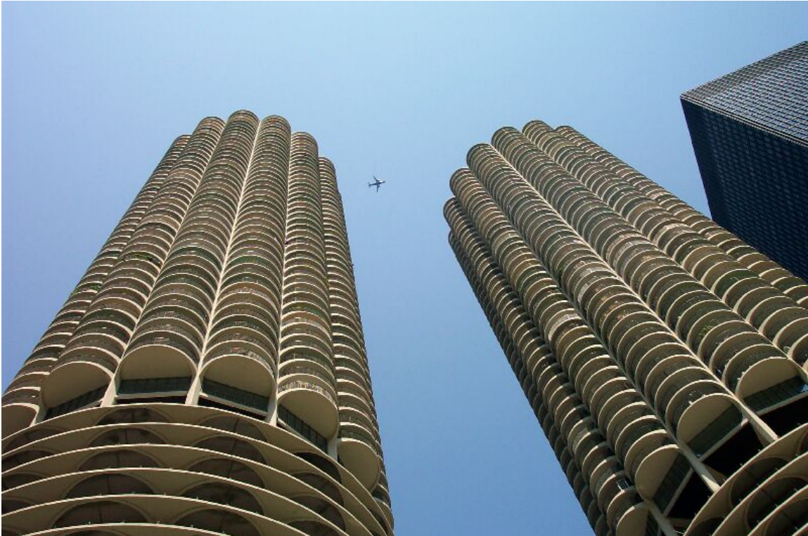
Figure 06: Marina City Fly Ash Structure in Chicago, IL Courtesy of: http://www.rmaiko.com/flyash.html
