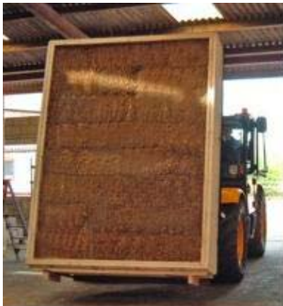
Figure 15: Modcell Precast Panel, Courtesy of: www.modcell.co.uk
